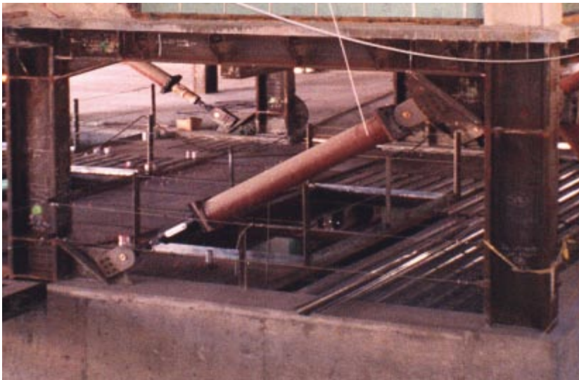
Figure 7: Diagonal Brace FVD Configuration
